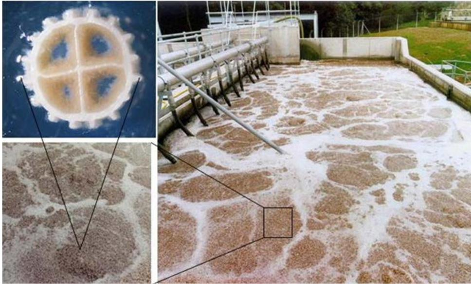
Fig. 4 The moving bed biofilm reactor (MBBR)
