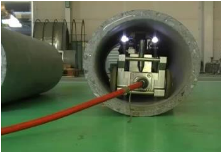
Not Deteriorated Pipe
