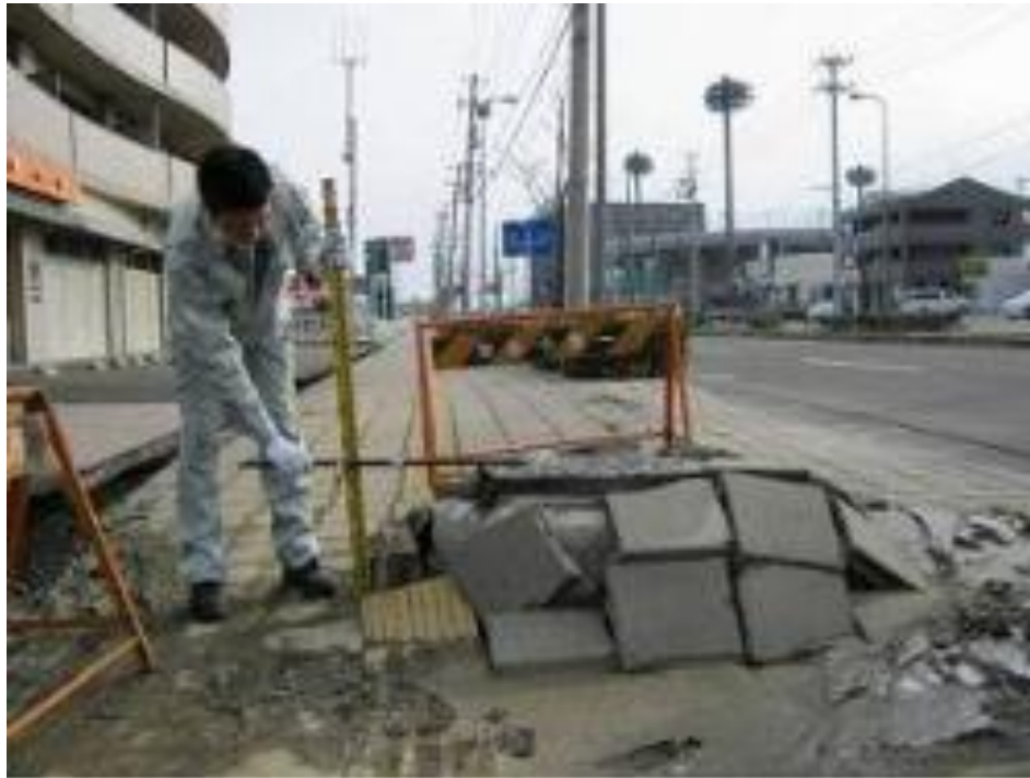
Manhole lifted by liquefaction
