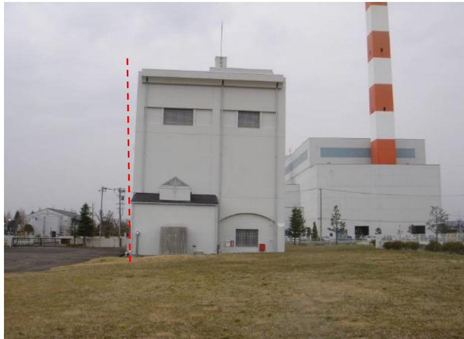
Inclined building by quake
