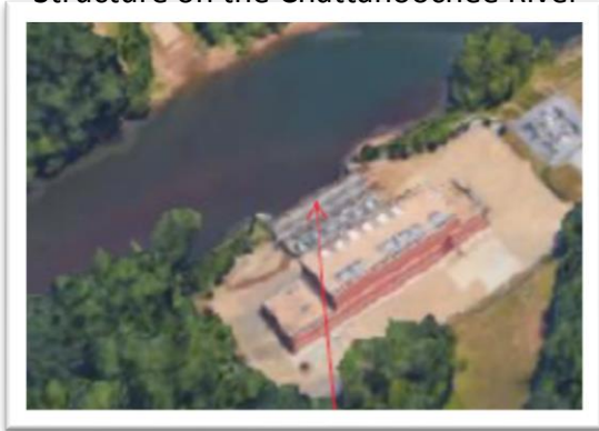
Figure 4. DeKalb County Intake Structure on the Chattahoochee River
