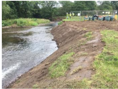
Washout chamber removed and bank reinstated
