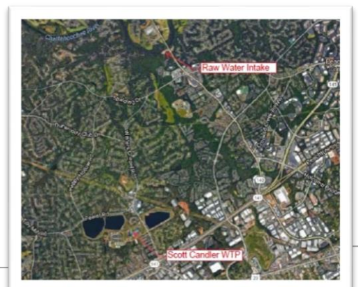
Figure 2. John A. Walker Pump Station and Scott Candler Water Treatment Plant
