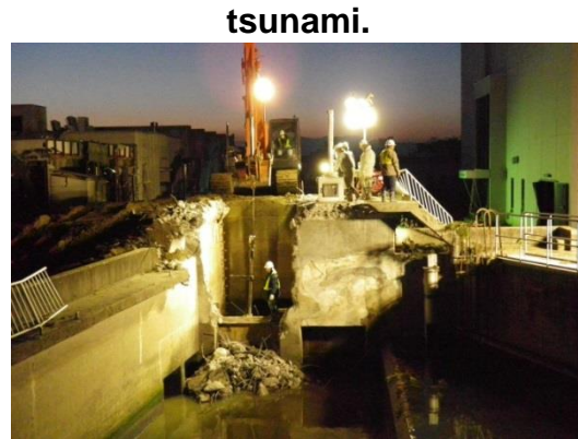
Picture 4.4: Breaking the emergency discharge gate of MGWWTP.
