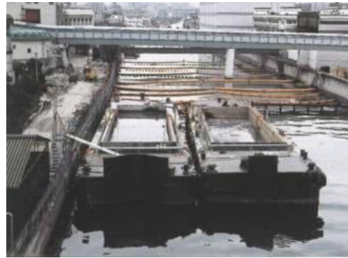
Fig.2 Temporary sedimentation tank using canal
