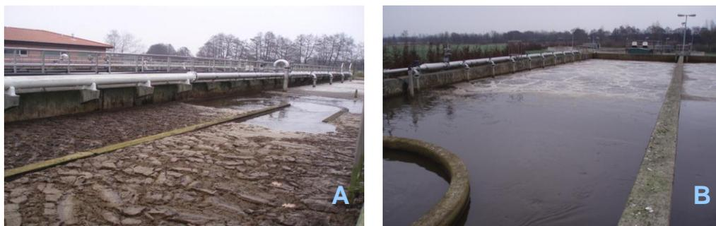
Figure 4: Activated sludge tanks of Seevetal WWTP during (A) conventional operation and (B) RAS-sonication.
