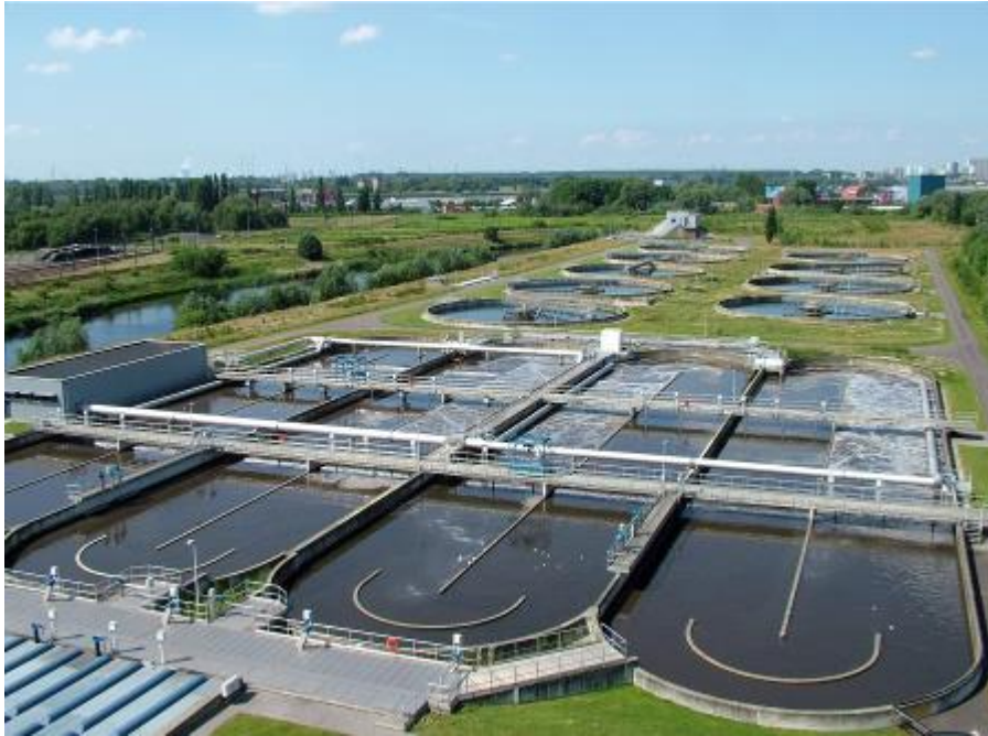
Waste water treatment plant Antwerpen-South (Belgium), source: Wikipedia NL edition
