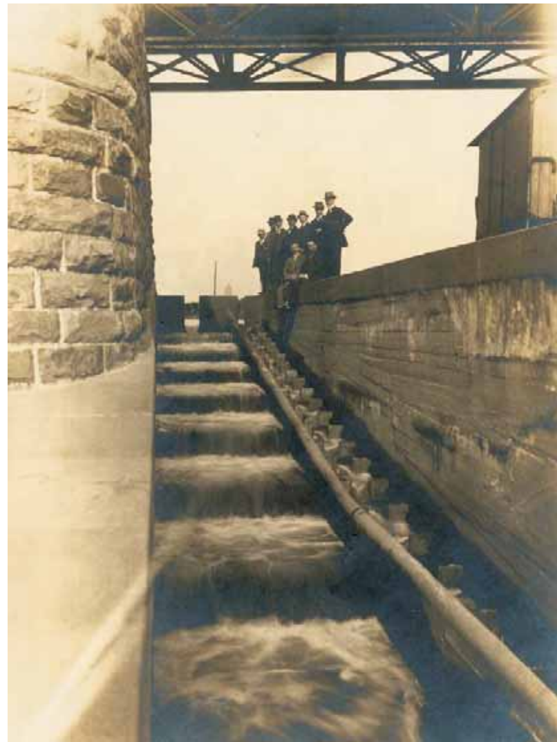
Figure 2: Pool-type fish pass Mülheim-Raffelberg/ Ruhr River (Germany) in 1920 (reference: Ruhrfischereigenossenschaft)
