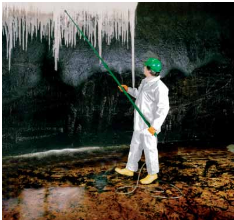
Disinfection cleaning of a water storage tank
