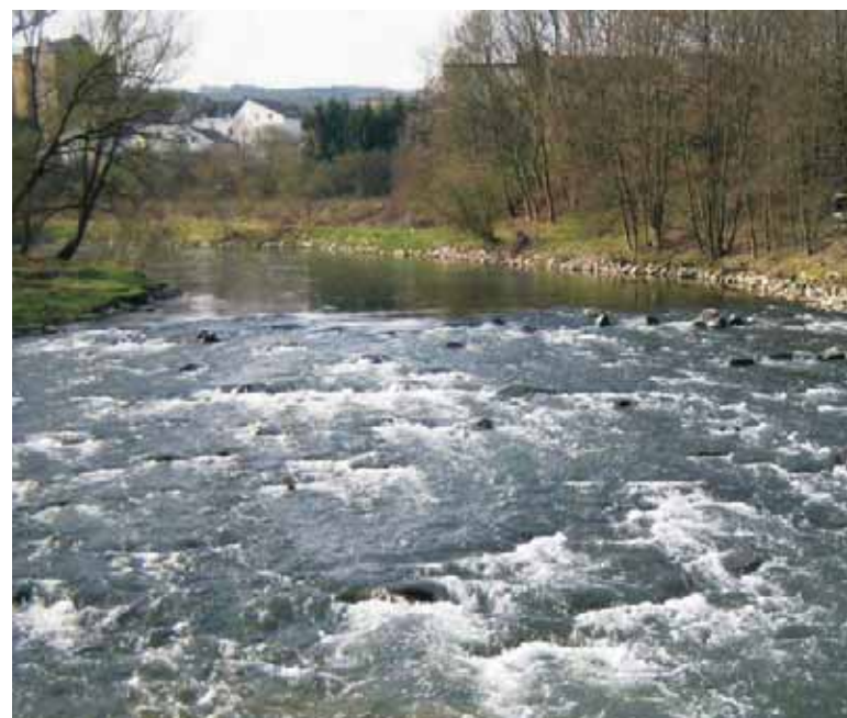
Figure 1: Rock-ramp fishway in Hüsten/Ruhr River (Germany)
