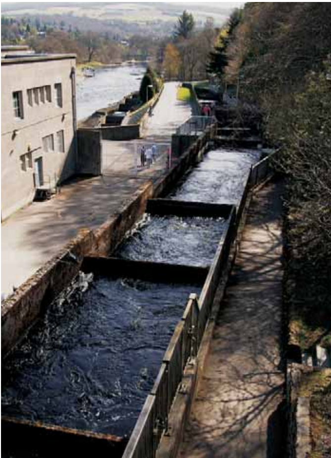
Figure 3: Technical pool-type fish pass Pitlochry Dam/River Tummel (Scotland)
